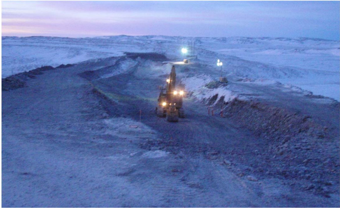
Photo 8: ~SSW view down key trench. Note excavator scratching/ removing 5/8” material in foreground.
