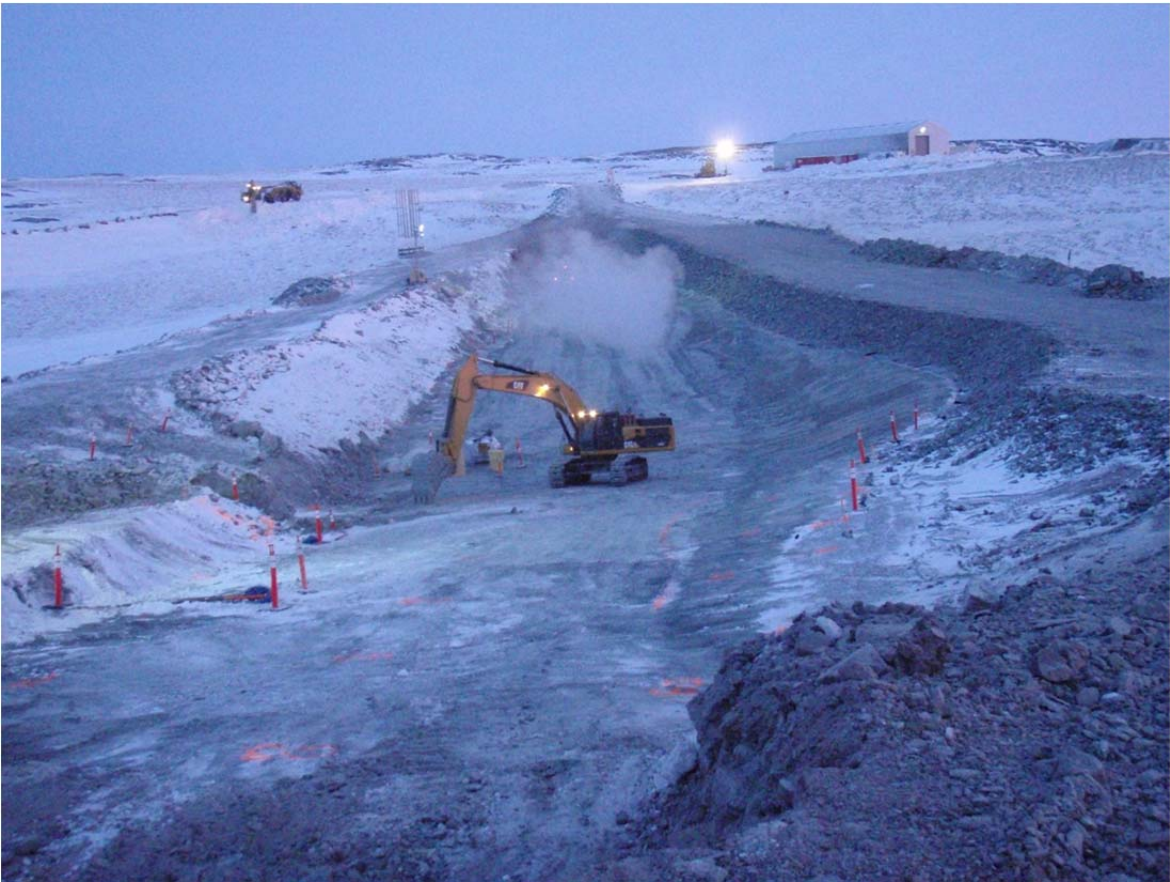
Photo 9: View of construction progress in the North Dam key trench, ~NE view down trench. Note the end dump piles of 5/8” material on the upstream of the dam.
