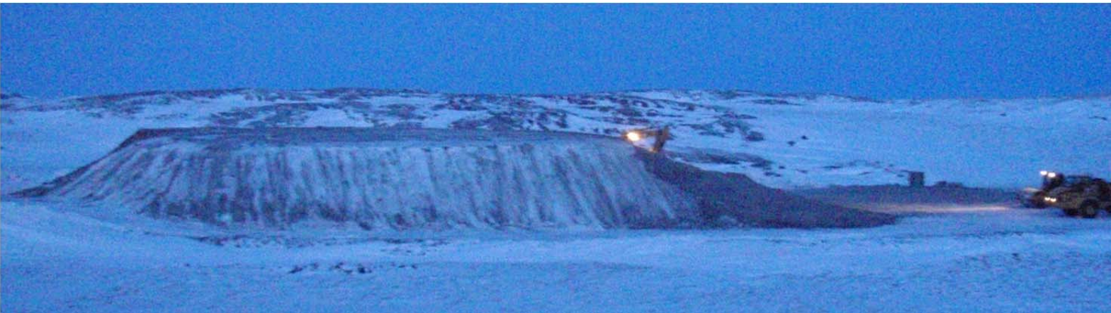
Photo 12 (bottom right): Excavator working on breaking/ mixing up frozen core material stockpile, ~NE view.
