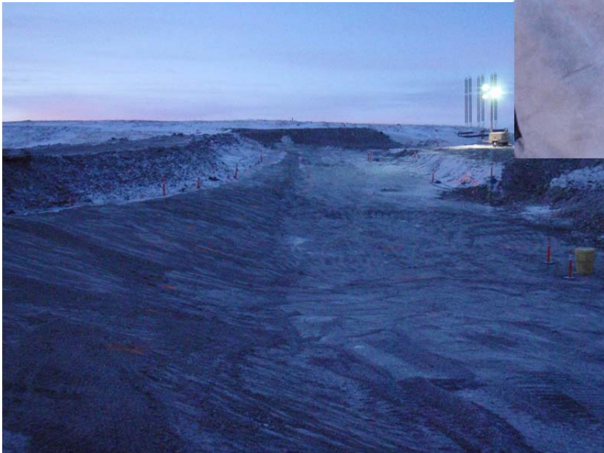
Photo 11 (mid left): Close up view of frozen 5/8” clear material being excavated in the North Dam key trench.
